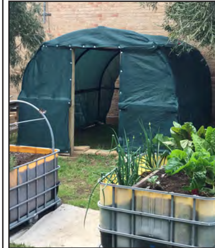
Progress with the shade house
