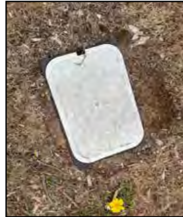
Hydrant cover with good access
