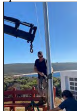
Hayden and Jamie bolting new flagpole into position
